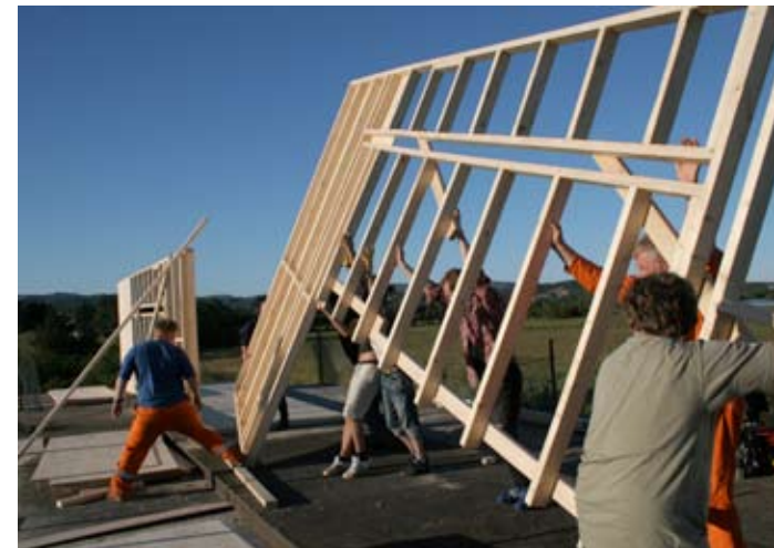
Feltstasjon Nesheim reises i god gammel dugnadsånd. Field station Neshaim is built by volunteers.
